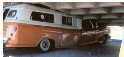
Hospital parking structure collapse crushes ambulance
