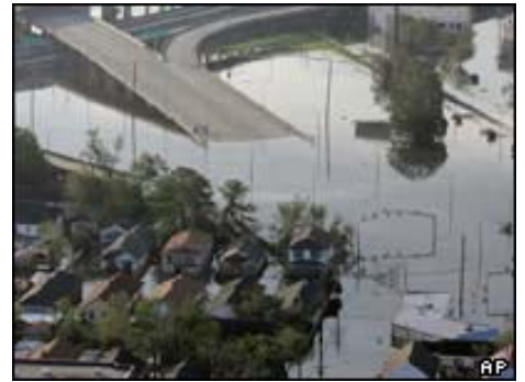
Roadways flooded in Hurricane
