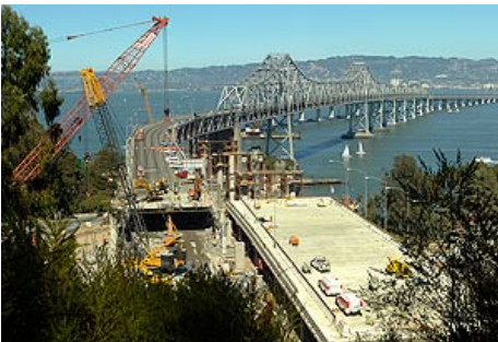
Bay Bridge deck replacement
