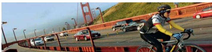
Golden Gate Bridge
