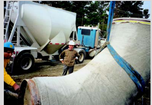
Pipe elbow being installed to avoid a landslide area
