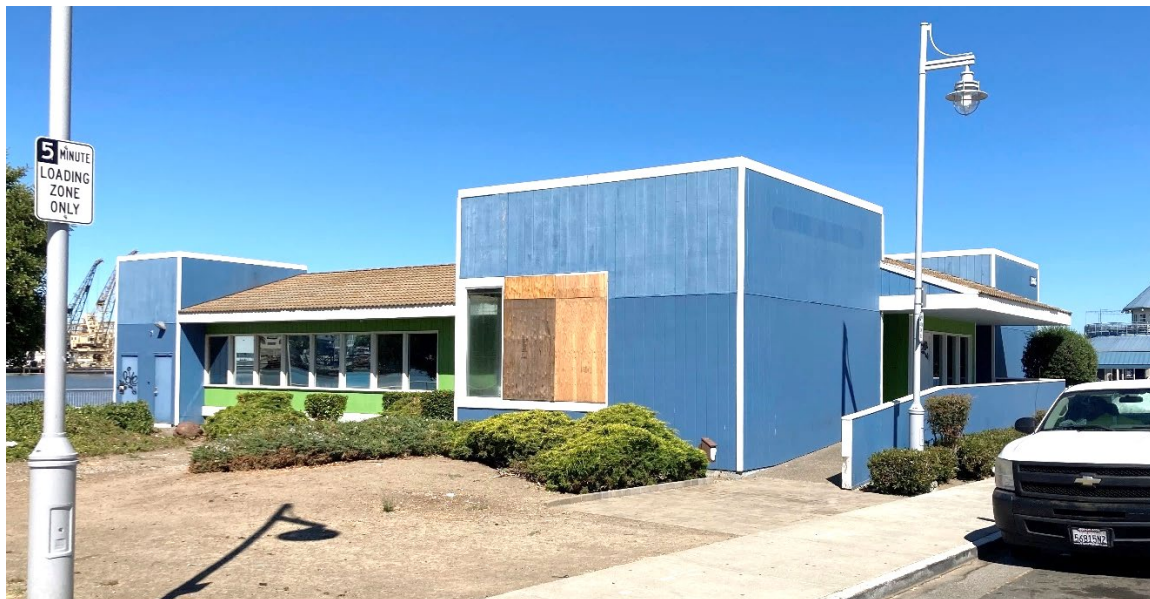
Southeast façade of 285 Mare Island Way. Source: ESA, 2023.
