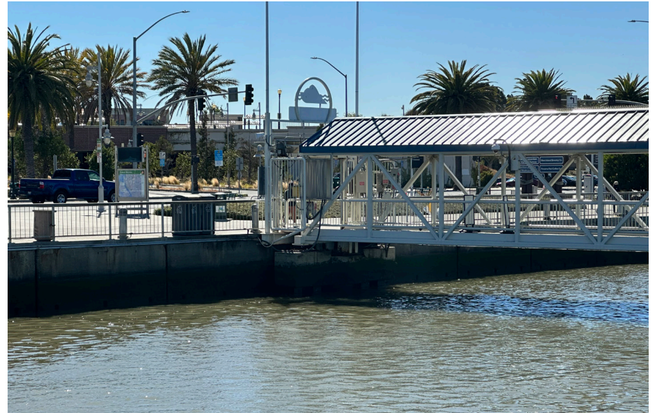
Access point and entrance gate to existing Vallejo Ferry Terminal gangway.
