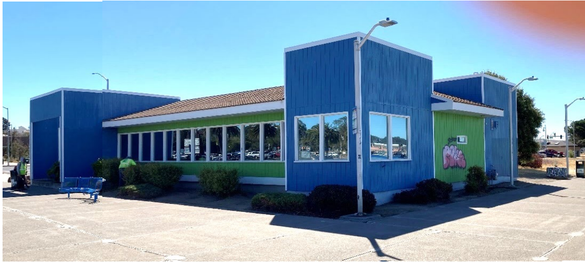
Northwest and southwest façades of 285 Mare Island Way. Source: ESA 2023.
