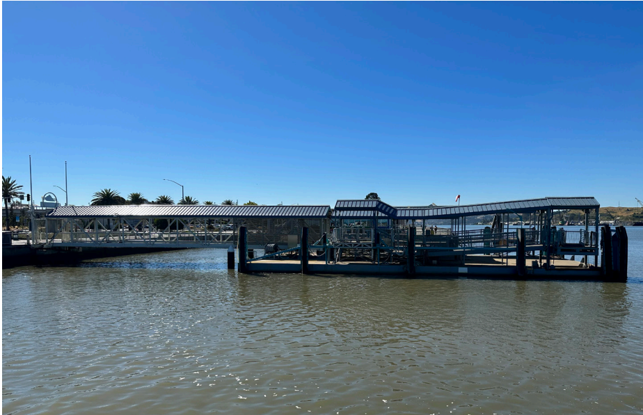
View of existing Vallejo Ferry Terminal facing south.
